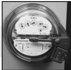
Electromechanical Meter Use Quick Install Guide or see section 5.2
